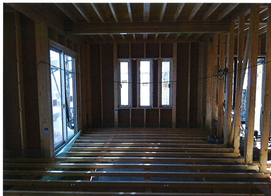
壁断熱施工前
